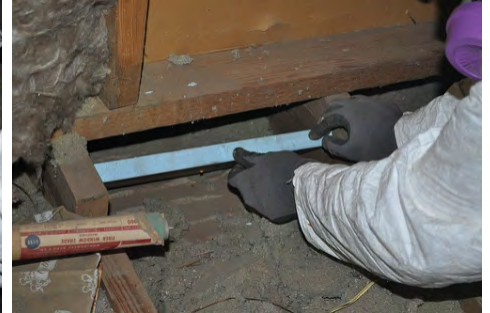
Align block with air barrier of conditioned space
