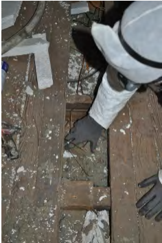
Check cavity for electrical junctions and penetrations
