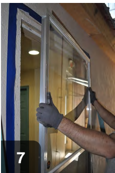
7 Remove window from rough opening
