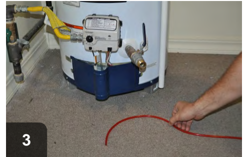
3 Place test hose by combustion appliance
