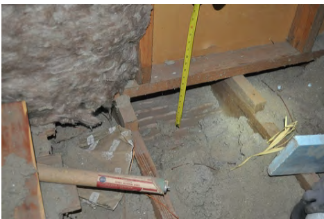
Bottom plates also need to be installed. Measure for size
