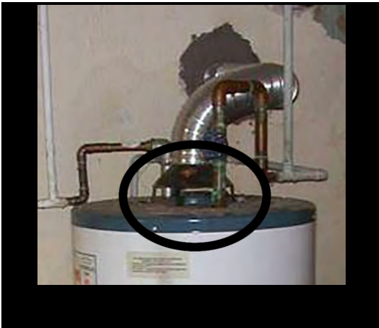
A natural draft water heater with indicative flue highlighted
