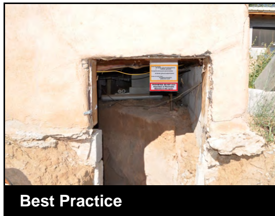
Sign should be highly-visible, securely-fastened, and durable
