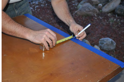
Measure and trim door, if necessary, to allow for door bottom
