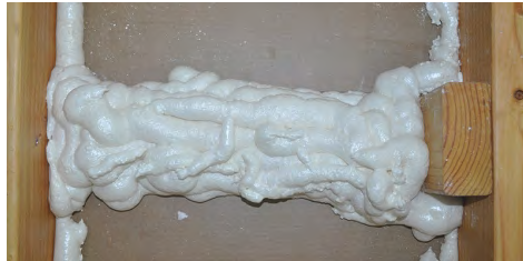
Option 2: Bridge cavities with spray foam
