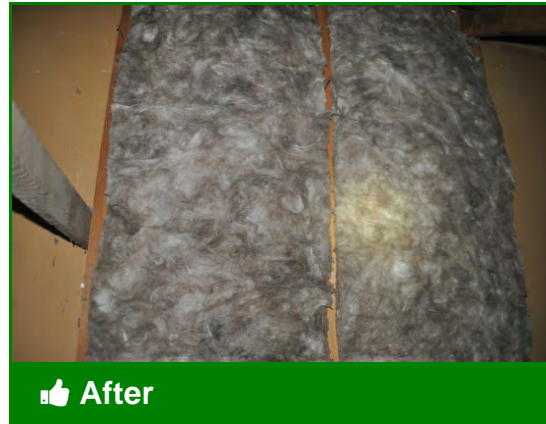
Properly fit insulation filling full volume of stud bay
