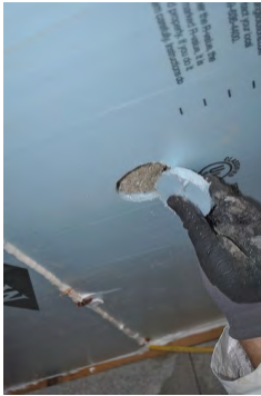
Once cavities have been filled to specified r-value, prepare plug
