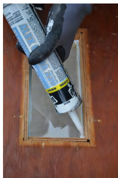
Seal glass into place from inside as well to ensure no air infiltration
