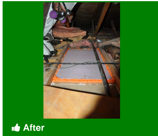
No gaps should remain after spray foam is applied
