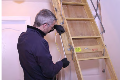
Weatherstrip around stair panel to encourage a tight seal
