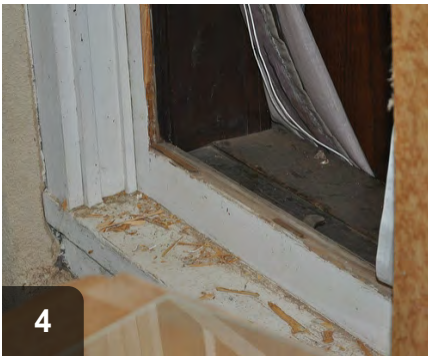
4 Use shims to center glass while installing push points
