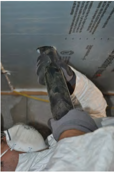
Fill cavities formed by rigid barrier with loose fill insulation
