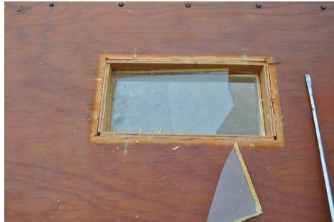
Remove broken glass and clean old sealant and glazing from rough opening
