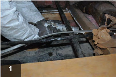
1 Caulk surrounding surfaces before setting cap in place
