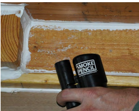
All Options: Test with smoke pencil to verify no air movement
