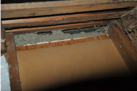
Knee walls missing top plates need one created from rigid material
