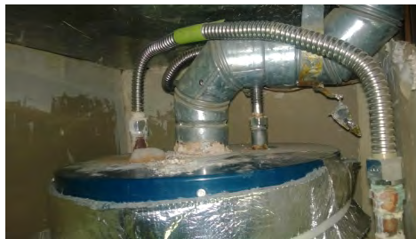
Inspect for missing draft diverter
