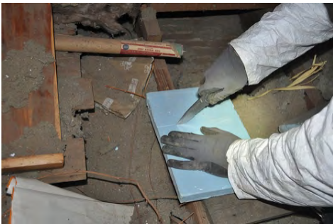
Bottom plate is cut to size
