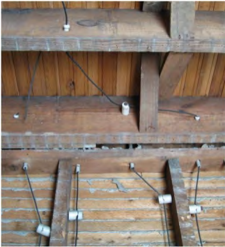
More knob & tube wiring
