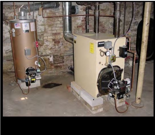
Check oil-fired furnaces and water heaters for proper fuel pressure
