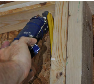
Seal penetration with caulk or fire-block, as appropriate
