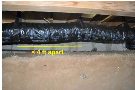
Flex ducts should have support straps at least every 4 feet
