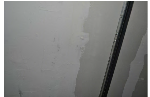
Tape and spackle access panel and test holes to repair garage ceiling
