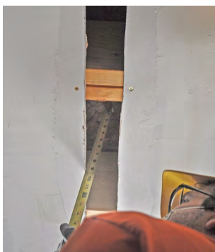
Measure joist cavity depth
