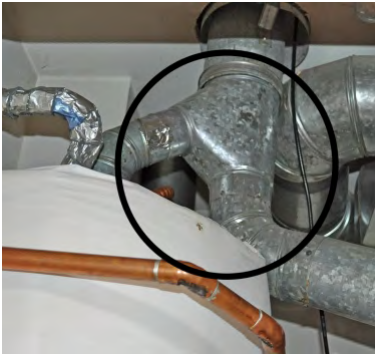
Common vent of natural draft appliances highlighted
