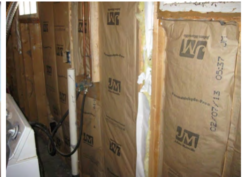
OR Kraft-faced fiberglass batts can be used with paper toward living space
