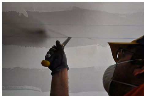
Cut through garage ceiling to access joist cavities below bonus room
