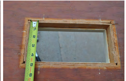
Measure rough opening and cut new glass to size
