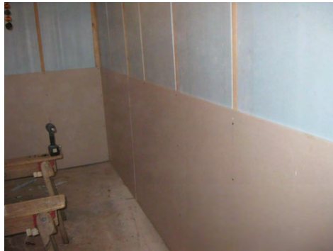
The drywall still provides an air barrier to keep moisture build up on wall
