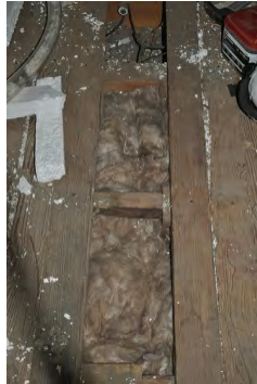
Fill entire volume of floor cavity
