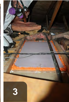
3 Additional sealant should fill in all remaining gaps after cap has been set
