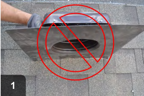
1 BAD: Termination fittings without collars should be avoided
