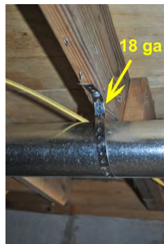
Metal strap should be at least 18 gauge and 1/2 inch wide
