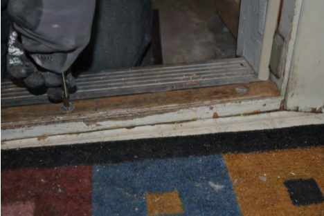
Adjust threshold to minimize gap and keep water out
