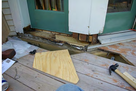
Once rotted materials are cut away, determine sizing of new materials
