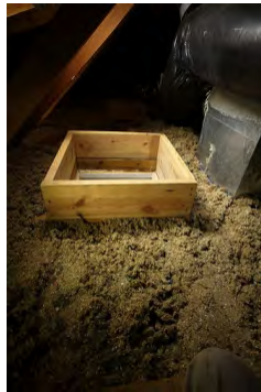
Build insulation dam from 3/4 inch lumber and seal around base
