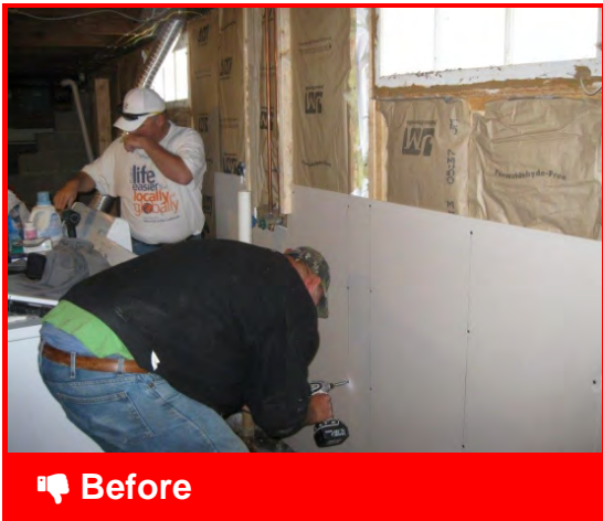
Kraft-faced fiberglass insulation is absorbent
