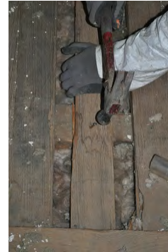
Once insulated, flooring should be reinstalled
