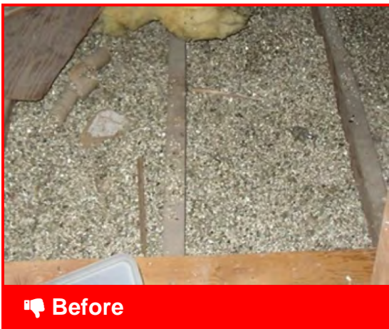
Material identified as vermiculite may contain asbestos
