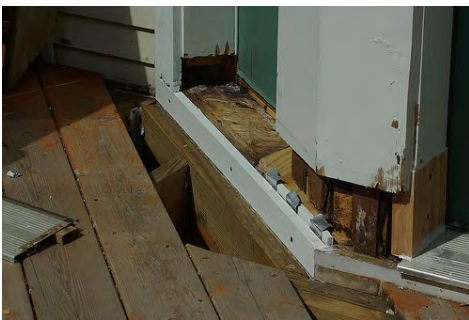
For exterior repairs, replace flashing
