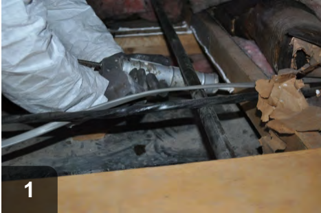
Caulk surrounding surfaces before setting cap in place
