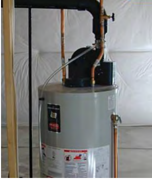
Power-vented water heater
