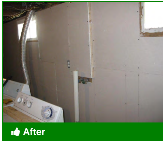
Drywall typically has a perm rating of 50--good for zones 1-6
