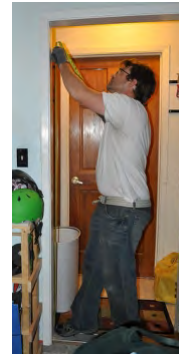
Measure doorway for weatherstripping
