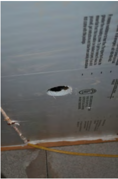
Drill hole slightly larger than nozzle into rigid barrier with hole saw
