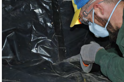
Tape (overlapped) floor seams to prevent movement and water leakage
