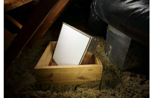
Weatherstrip around bottom edge of hatch cover to create air tight seal
