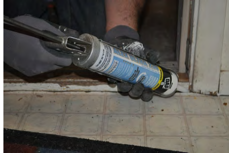
Caulk along threshold from inside and outside to prevent water infiltration
