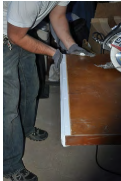
Ensure door bottom fits snugly around door and fasten into place
