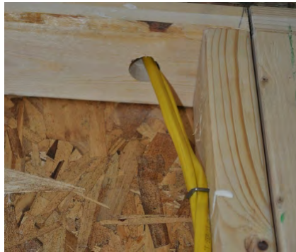
Penetrations and bypasses should be sealed to keep insulation in cavities
