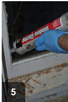
5 With push points in place, glaze to air seal new glass pane in sash
