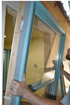
Flanges have been folded out to allow for easy installation
