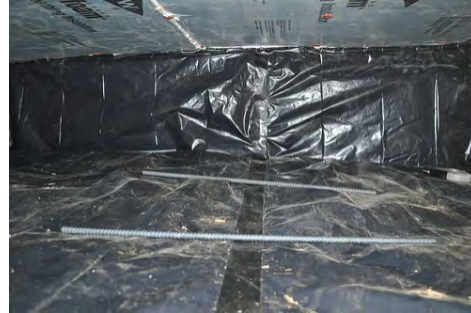
Ballast or fasteners can hold barrier in place securely
