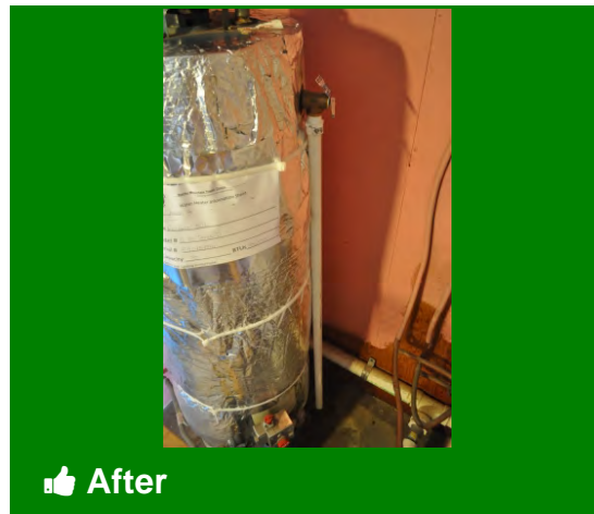
T&P discharge should be piped to a safe and observable location
