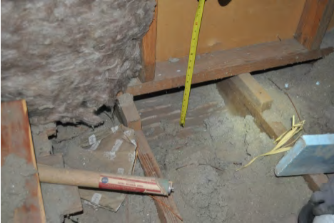
Measure floor cavity for new bottom plate
