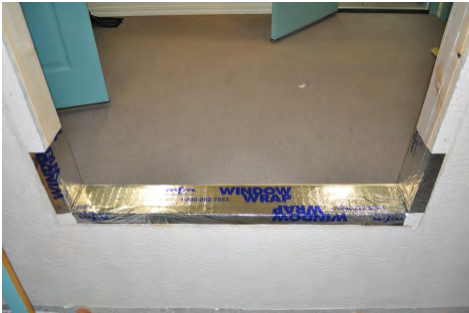
Install flashing to manufacturer specs and industry standards
