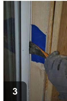
3 Remove stops while attempting to keep damage to rough opening to minimum
