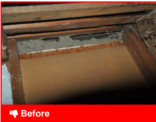
Top plate is missing from knee wall
