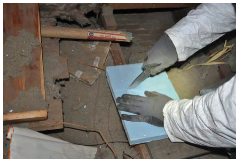
Cut to size and attempt to install in line with air barrier above
