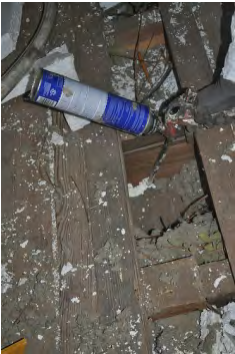
Air seal any penetrations
