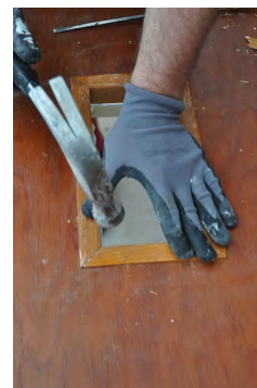
Replace stops and rehang door
