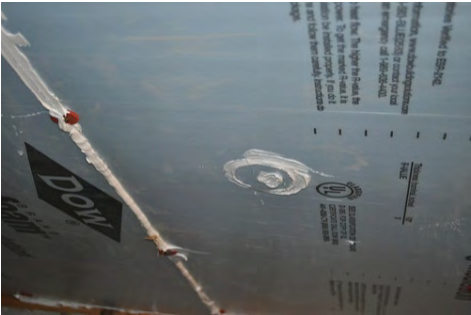
Securely seal plug into rigid barrier to prevent leakage
