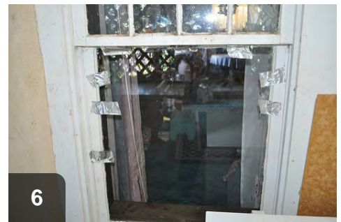
6 Secure pane in place with tape to hold until glazing sets
