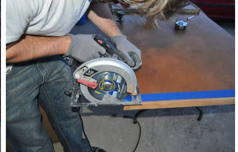
Trimming to allow for door bottom
