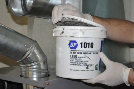
GOOD: Wear nitrile gloves when handling mastic
