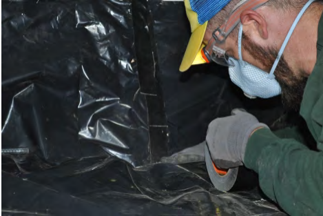
Seams can be taped to prevent water leakage
