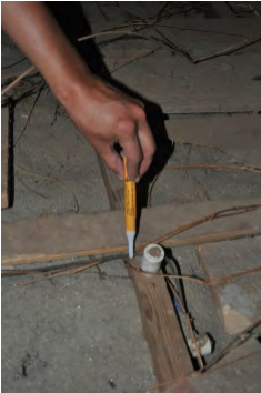
The entire knob and tube system should be disabled
