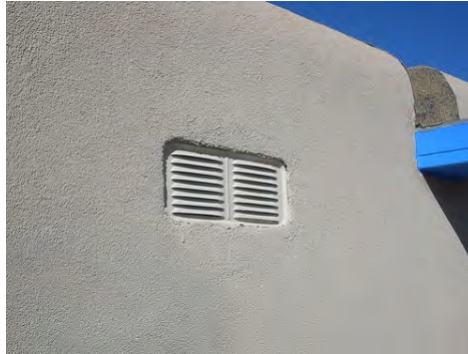
Vents in the space below the roof help maintain proper air flow
