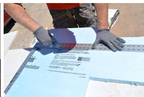
Cut XPS, or other rigid material, to measured size of joist cavity
