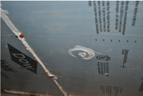
Seal rigid barrier to prevent leakage
