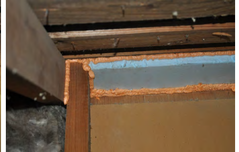
New top plate should be sealed to surrounding joists and studs
