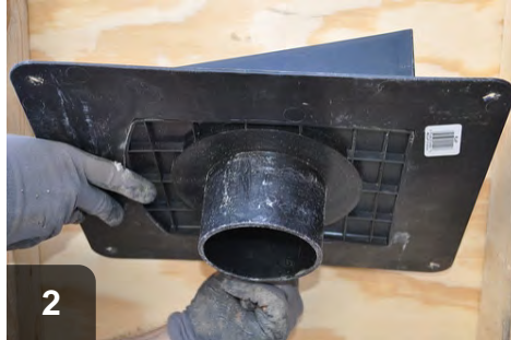
2 Termination fittings with collars should be used for exhaust ventilation
