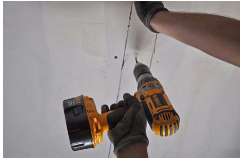
Close cavities with access panel cut out at the beginning
