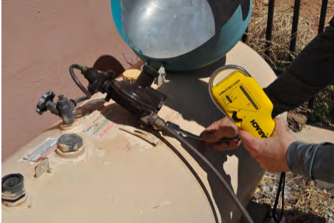
Check all raw fuel lines for leaks
