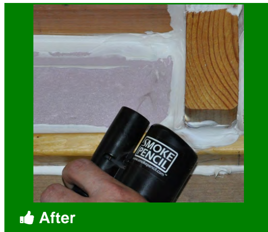
Whatever option chosen, test for visible air movement with smoke pencil
