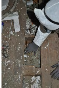
Check cavity for electrical junctions and penetrations
