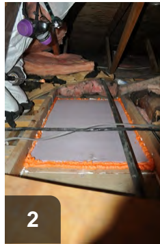
Use sealant to fill all remaining gaps
