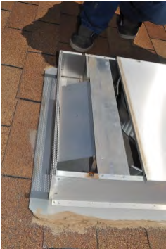
Backdraft damper on roof mounted exhaust fan
