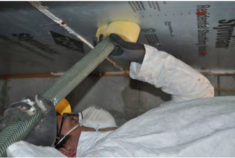
Dense pack insulation into floor cavities
