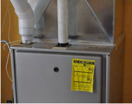
Two-pipe 90% efficiency furnace
