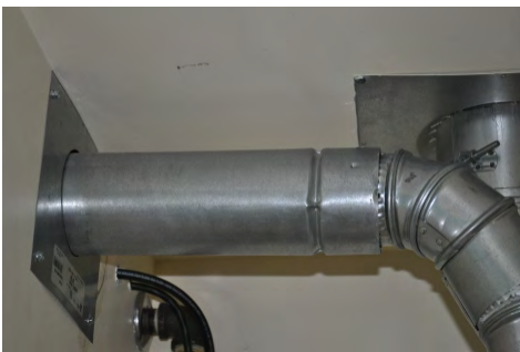
Inspect ventilation systems for inadequate slope
