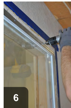
6 Remove exterior fasteners to free window
