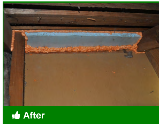
New top plate is sealed to adjacent framing
