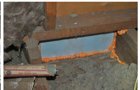
Seal to surrounding joist
