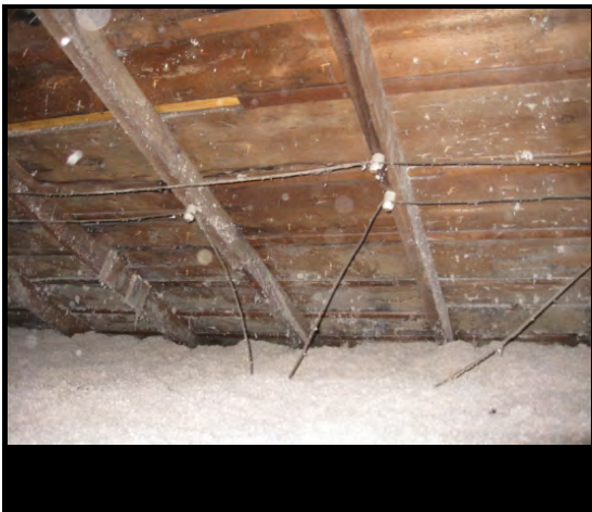
Knob and tube wiring should be identified before work begins
