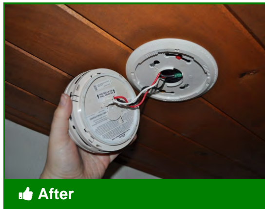
Installation of hard-wired smoke alarm
