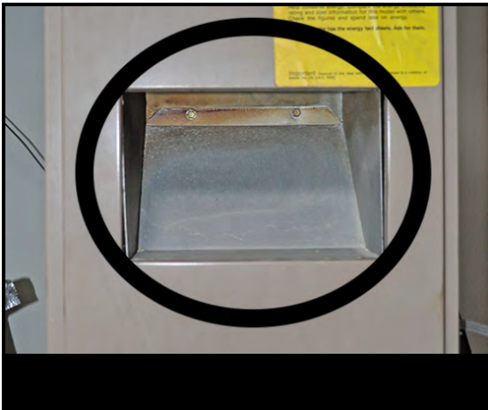
Category I 70% efficiency gas furnace with intake vent highlighted
