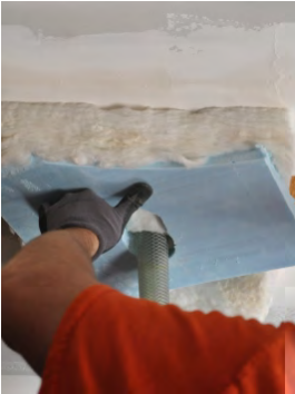
Blow insulation into cavities to density appropriate for chosen material
