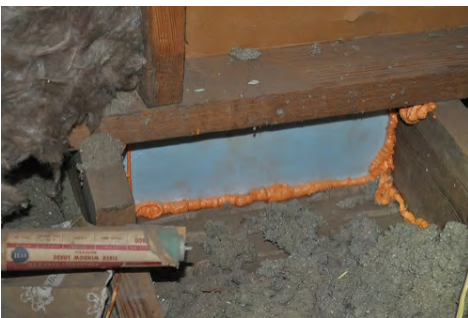
Air seal around new bottom plate with spray foam
