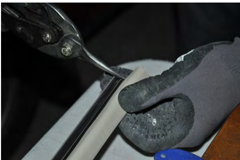
Notch upper ends of side weatherstripping to allow for top piece
