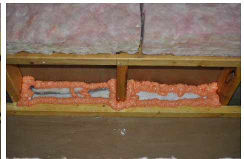
Option 4: Bridge cavities at new ceiling level with wrapped batts and SPF
