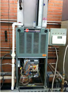
Cat I 80% efficiency furnace
