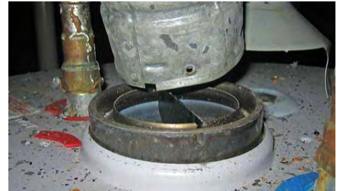
Inspect ventilation systems for disconnected pipes
