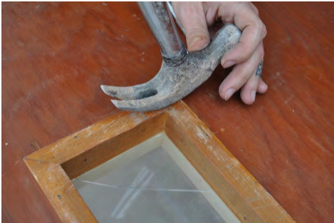
Remove stops, taking care not to damage them
