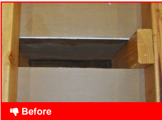
Wall cavities are open to attic
