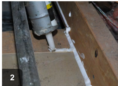
2 Sealant should extend along surround joist and into seams at top plates
