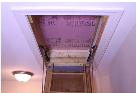
Insulation and sealing should be airtight but openable
