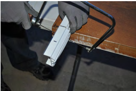
Cut door bottom to width of door
