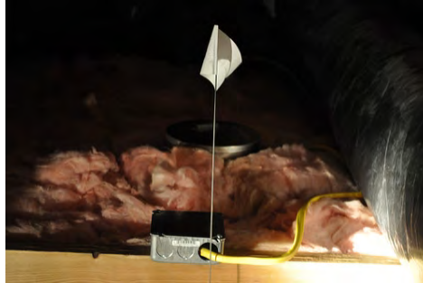
Flag and install covers on electrical junctions
