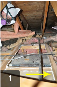
Caulk along all joists before setting cap
