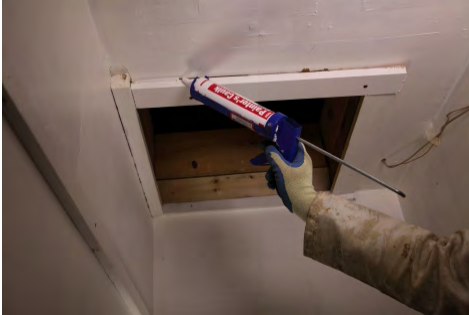
Remember to seal around finish details and framing on interior
