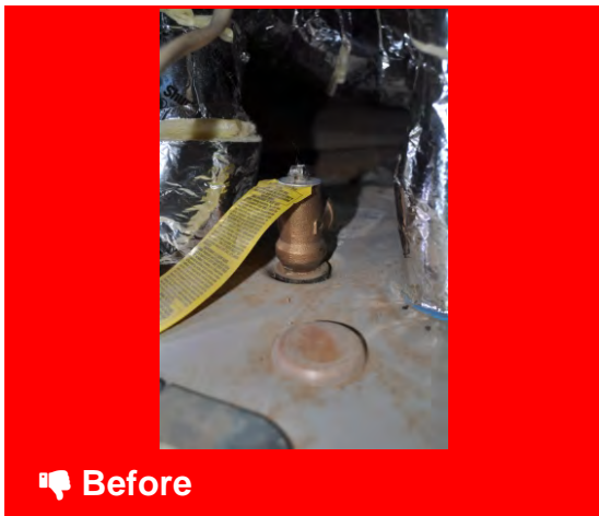
Water heaters should be not capped off at t&p valve
