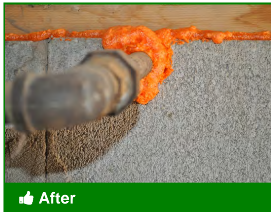
Sealed with durable material to prevent air and water leakage, and pests
