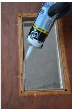
Apply sealant to rough opening and place new glass
