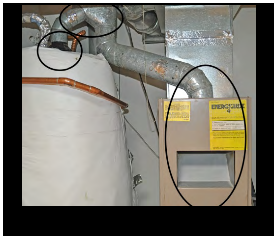
Natural draft water heater and natural draft furnace with common vent
