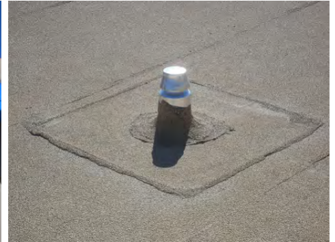
Mushroom capped vents in the roof are equally important to air flow
