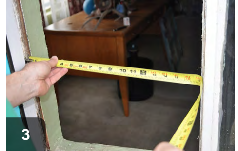
3 Cut replacement glass 1/8" smaller than measured opening
