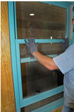
With window secured in place, check for proper function
