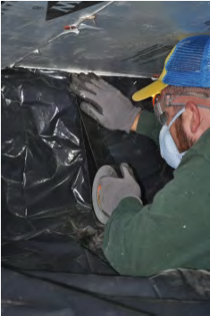
Tape wall seams and press to ensure airtight bonding of adhesive
