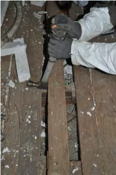
Pry up flooring to access floor cavities
