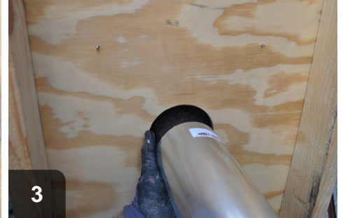
3 Collared fittings extend through the roof to fasten securely with duct
