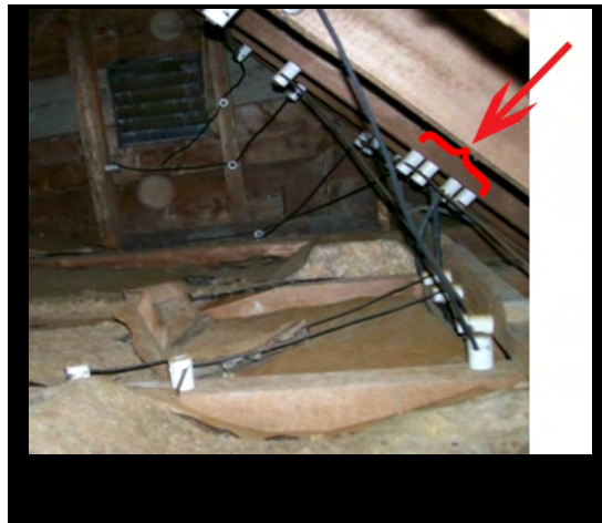
Distinctive "knobs" are highlighted. This wiring can be a safety hazard
