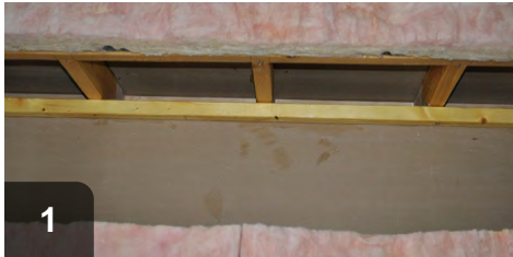
1 Soffits open to the attic need to be sealed to maintain air barrier
