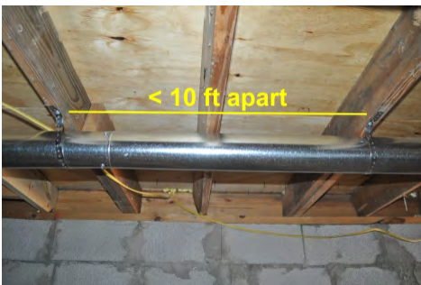
Metal ducts should be supported at 10 feet or less with wire or metal strap
