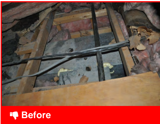
Dropped soffits need to be capped and sealed to prevent leakage
