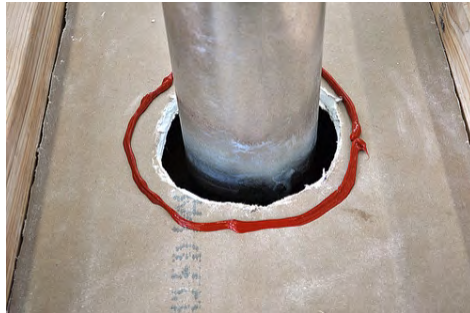
High temperature caulk should be used for flues and chimneys
