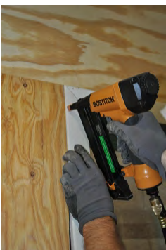
Prime and replace interior trim and, if needed, sill
