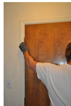
Rehang door and verify fit, operation, and lack of air infiltration
