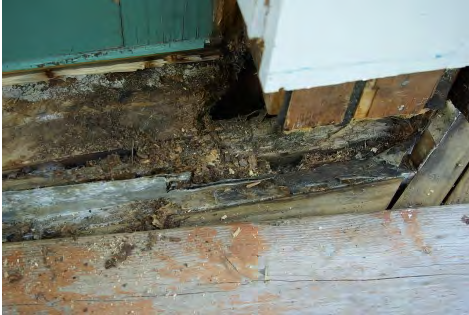
Remove sill to determine full extent of rot and necessary repairs
