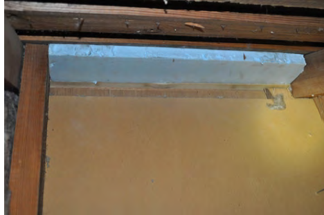
Top plate holds dense pack insulation in cavity
