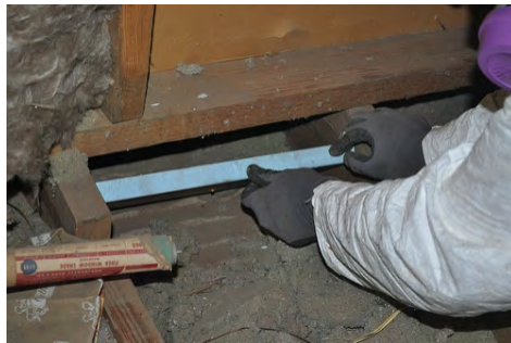
Bottom plate is placed in line with interior air barrier
