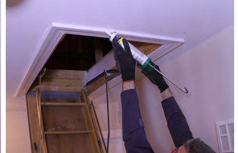
Remember to seal finish details and trim
