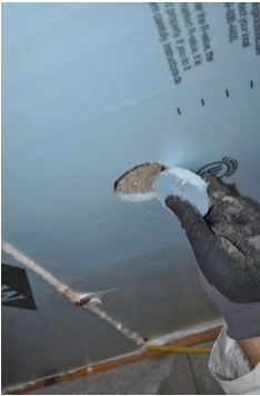
Once cavity is filled, prepare plug to reseal rigid barrier
