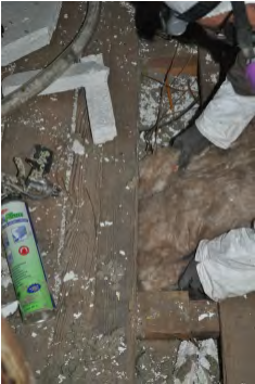
Insert fiberglass batts into floor cavities, kraft-face down
