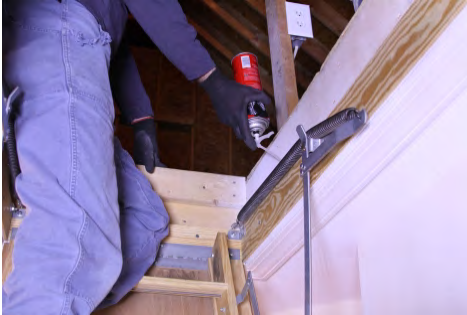
Seal around frame of pull-down stairs with appropriate sealant
