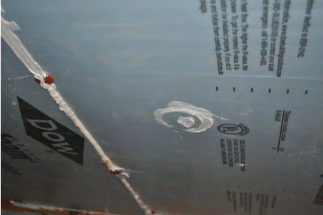
Plug access hole and seal to maintain air barrier
