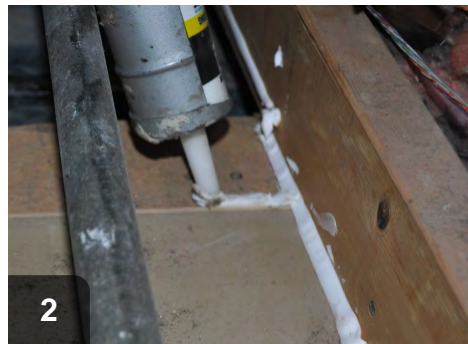
Sealant should extend along surround joist and into seams at top plates
