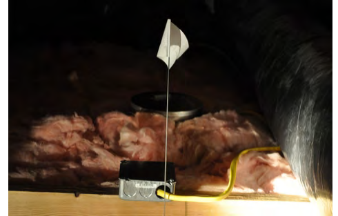
If electrical junctions are found, they should be enclosed and flagged
