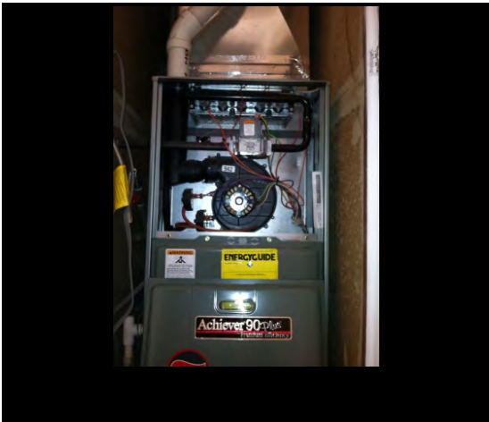
Single-pipe 90% efficiency furnace with forced draft
